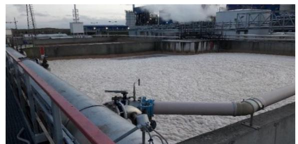
Fig. 7 Aerotanks – part of the biological cleaning equipment for wastewater
