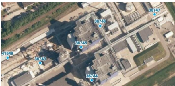
Fig. 9. Boreholes for the underground water monitoring
