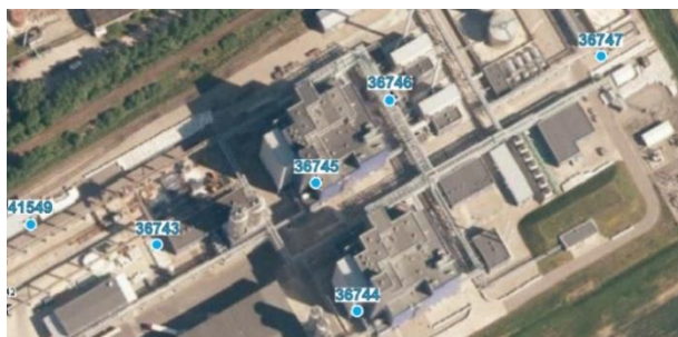
Fig. 9. Boreholes for the underground water monitoring
