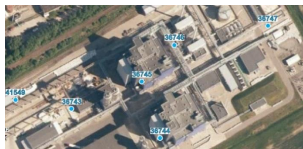
Fig. 9. Boreholes for the underground water monitoring
